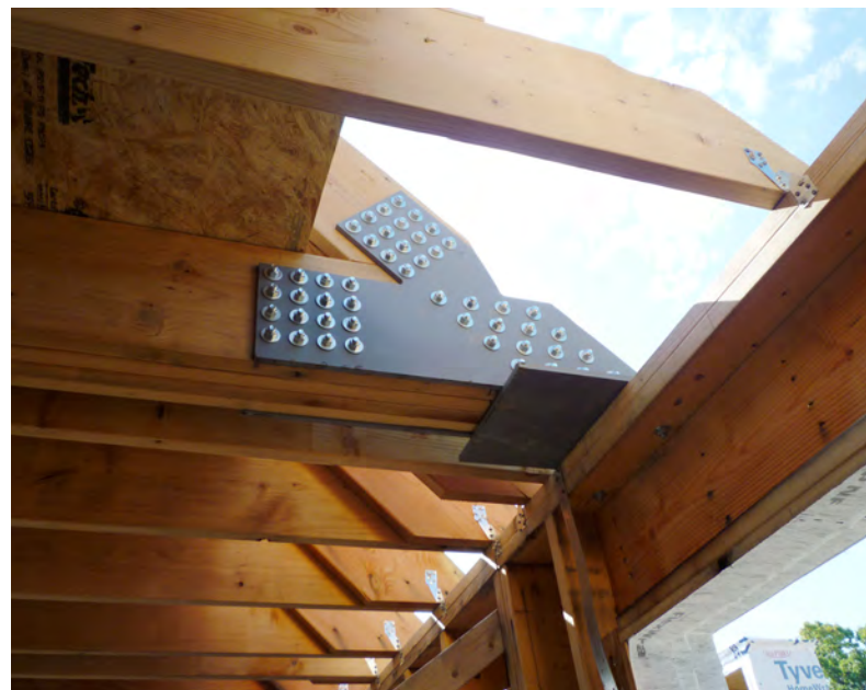
Figure 3 – Custom wood to wood connector
