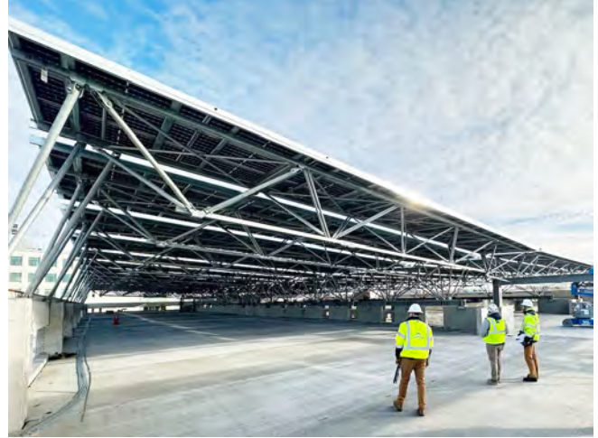
A large carport system in construction atop a parking garage
