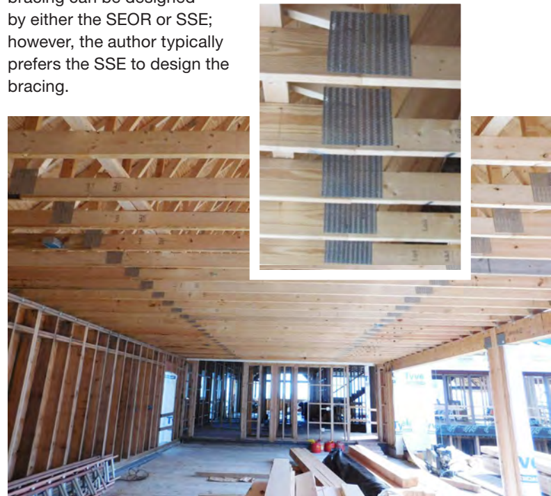
Figure 1 - Metal plate connected wood trusses and punched sheet metal plate connectors
