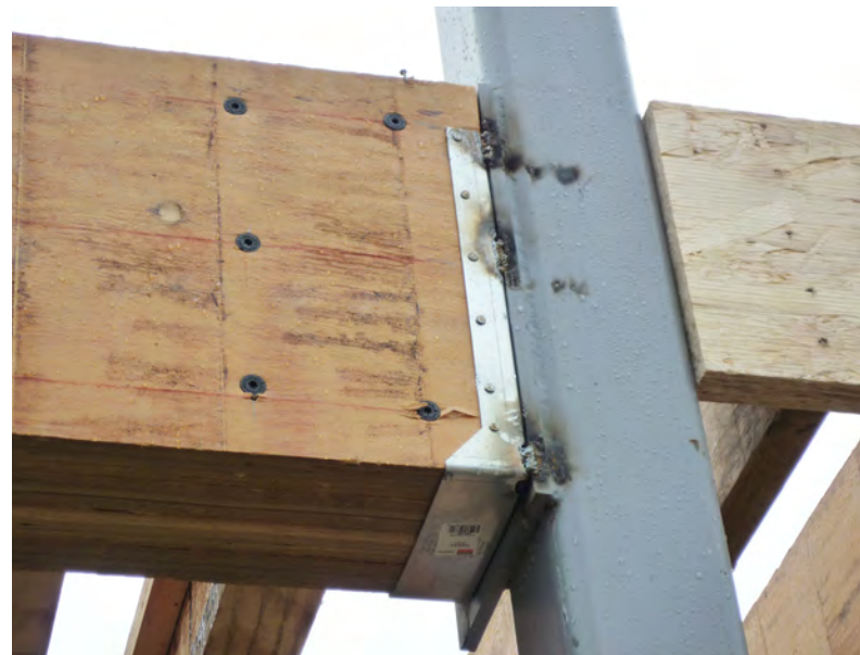
Figure 5 – LVL Connection to Steel Column
