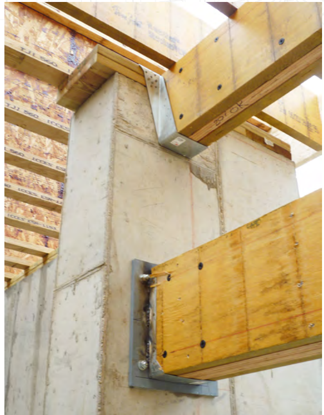
Figure 7 - Custom wood connection at concrete wall
