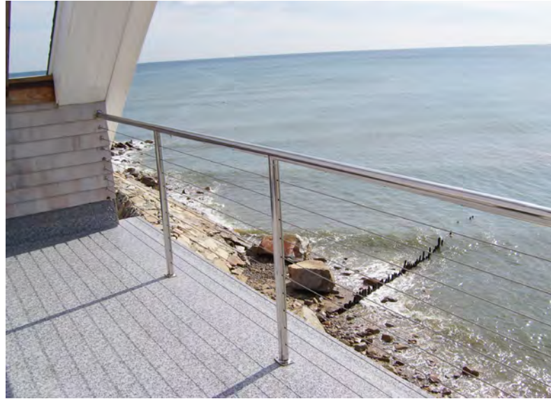
Stainless steel is a corrosion resistant iron alloy that contains chromium and other elements making it particularly well suited for salt water and other environments
