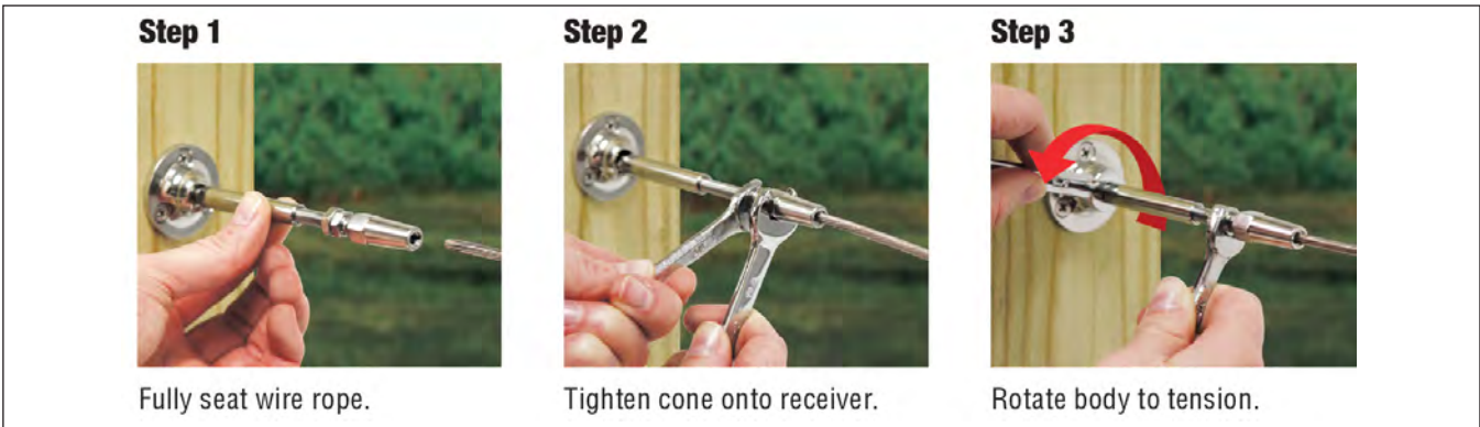
Mechanical connection of cables to posts relies on specialty hardware and common hand tools and is often used for surface-mount systems
