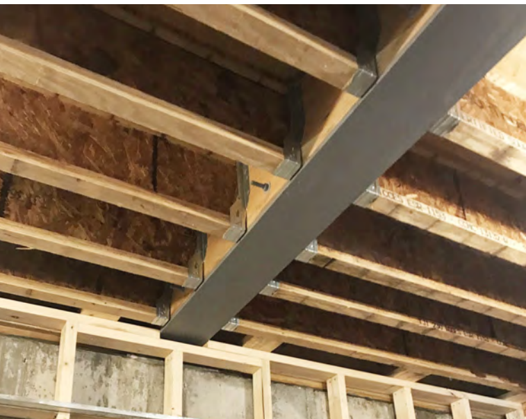
Figure 4 - Wood joist connection at steel beam
