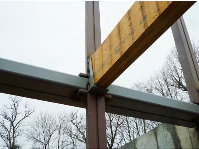
Figure 6 – Custom steel connector to column
