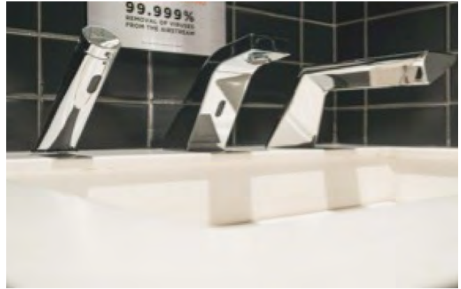
Figure 3. The integration of soap, water, and a dryer in one assembly impressed Andy Yee, principal managing partner of Bean Restaurant Group
