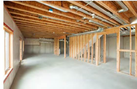
Concrete, even after curing, continues to release moisture and interact with the ambient relative humidity. For this reason, it's especially important to monitor concrete RH levels
