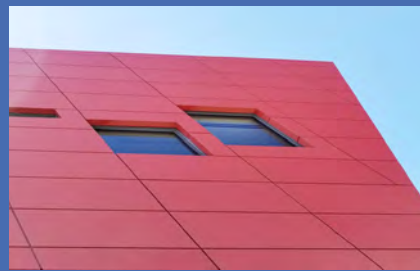
Chicago’s Esperanza Health Center features an MCM exterior with a prismatic finish
