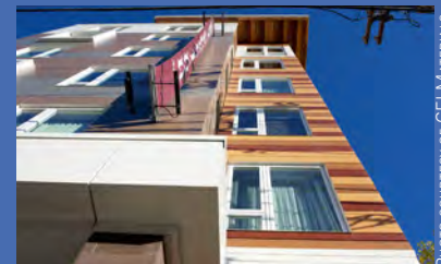
Shown is the MCM exterior and faux wood finish of the Marriott Residence Inn located in Watertown, Massachusetts
